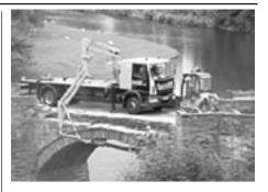
Work on Pont Carrog proceeding with the aid of the 'cherry picker'. The picture also reveals the original bed of the roadway and the immense thickness of tarmacadam which has built up over the years.
